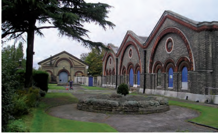
Garden terrace with workshop at far end
