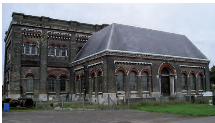
Beam Engine House and Triple Expansion Engine House
