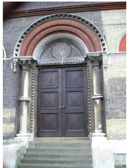
Side entrance to Beam Engine House
