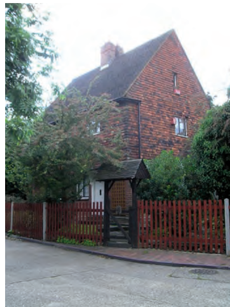
15 Old Forge Way from Rectory Lane
