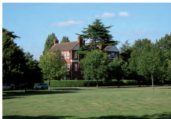
View to original 'boys house' across the open space
