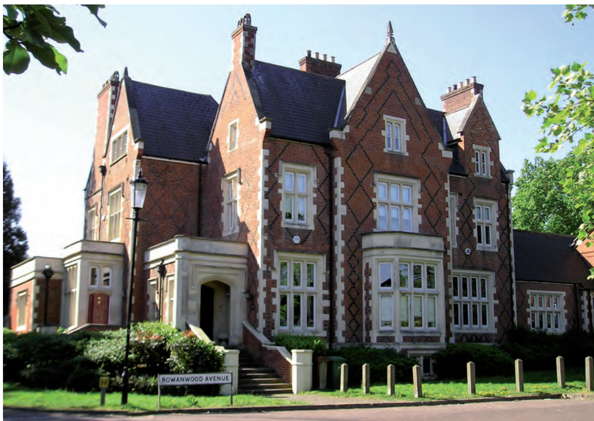
The Hollies, built as a Victorian country home in 1854, formed the administrative centre for the Greenwich Poor Law Union's 'model home for orphans', opened in 1902. [Renamed The Manor House when site redeveloped.]
