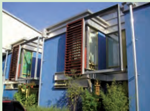
Sun screens, Greenwich Millennium Village
