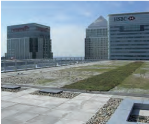
Green roof, Barclays Bank, London
