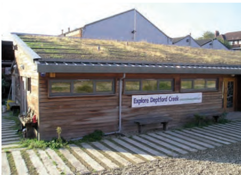
Green roof and water collection, Creekside, Deptford
