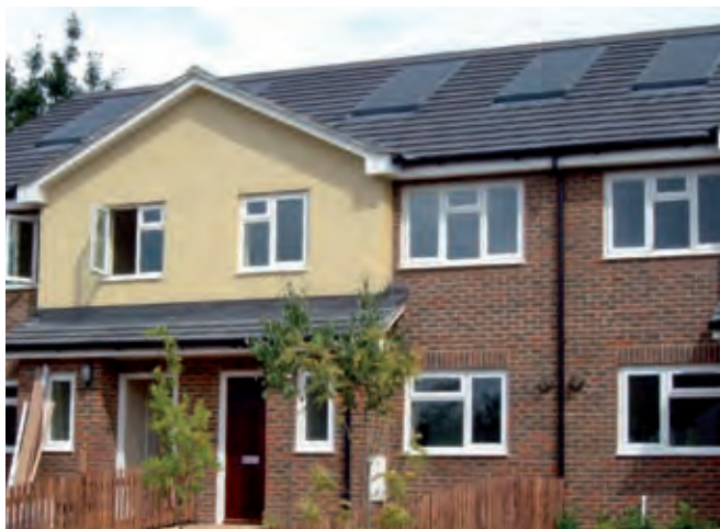
Above: Solar thermal tiles
