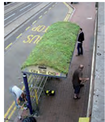
Green roof bus shelter, Sheffield
