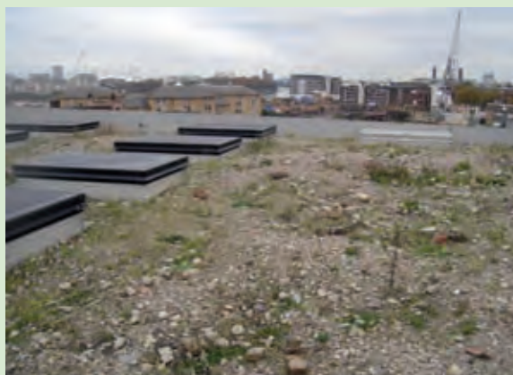
Brown roof, Laban Centre, Deptford
