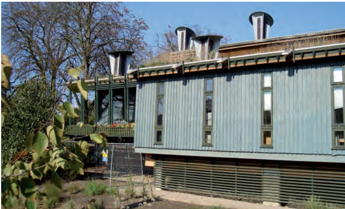
Passive stack ventilation, Horniman Museum, Forest Hill
