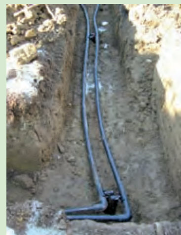
Ground works for ground source heating
