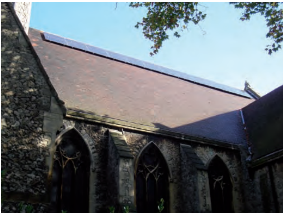
Photovoltaics, St. Peter's church, Brockley
