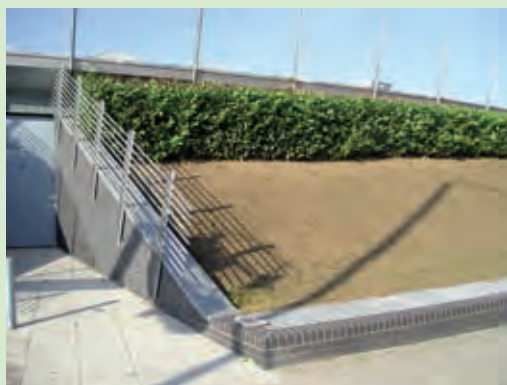
Earth walls, Greenwich Peninsula
