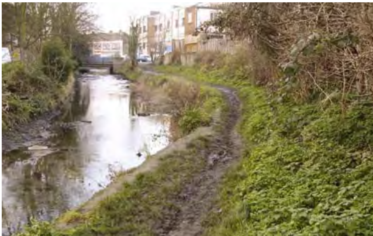
Footpath 106, showing a section of the footpath next to the River Cray before improvement
