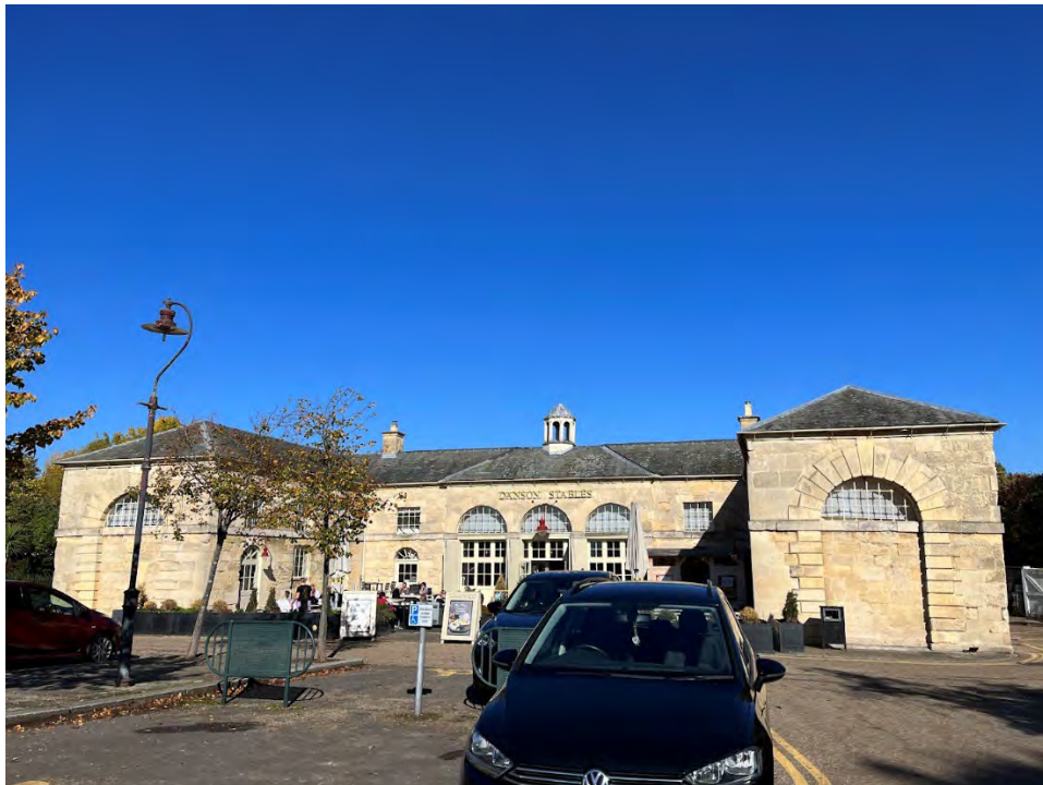
Plate 6 View of southern elevation of the grade II* listed stable block
