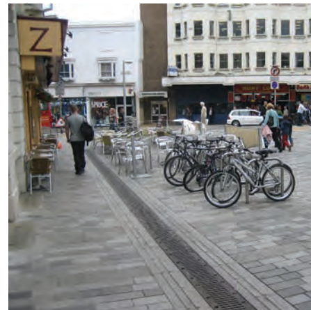
The photos illustrate examples of successful shared surfaces in the centre of Brighton
