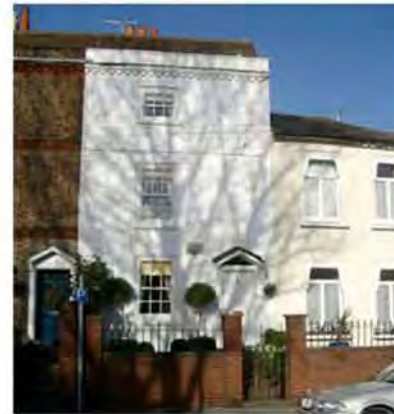
Existing Crayford building character
