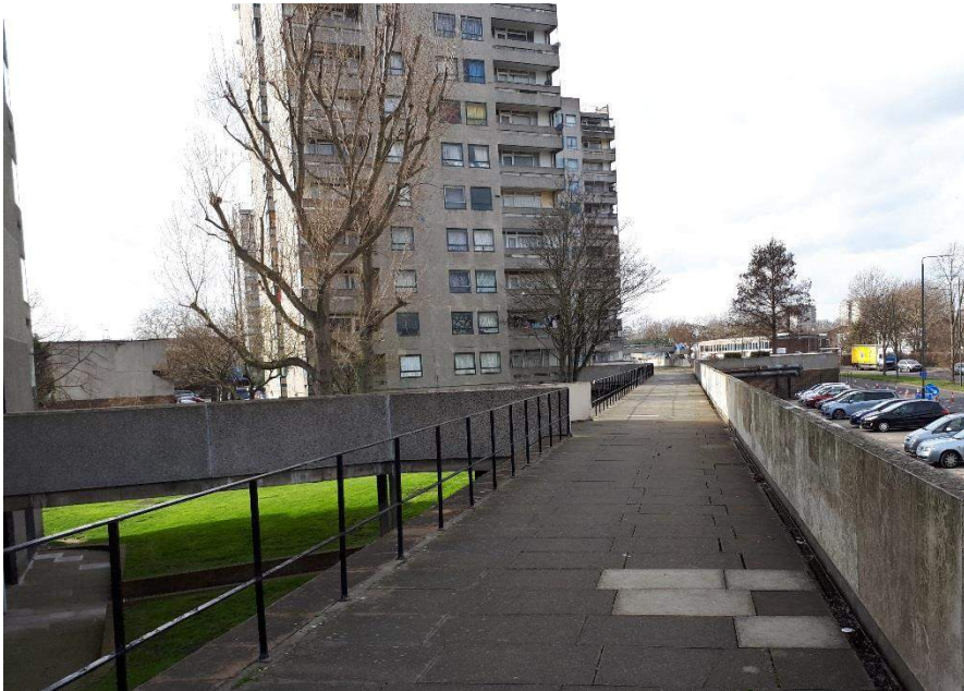
Figure 13: Parkview flats viewed from podium walkway
