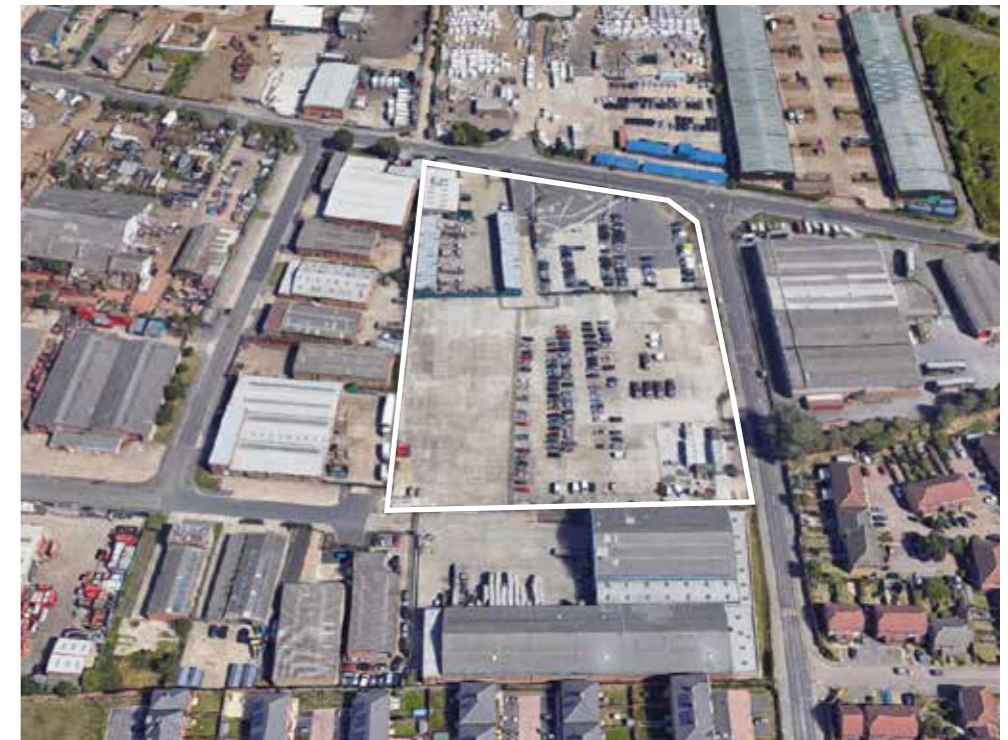
Erith Speedy Erith Site ID - 162 Site Area - 1.87 Ha Building Condition - Average/Poor
