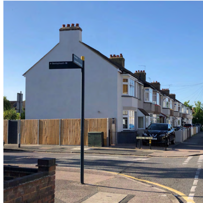
Fig.95 Generally new signs should use an established system to avoid confusion, such as those contained in the Traffic Signs Manual (mandatory for highway areas) or wayfinding similar to Legible London in town centres or near stations. Information included on directional signs should be specific and suitable for the needs of the intended user.
