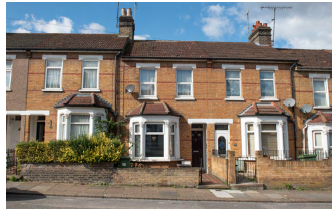
■ The dense terraced typology is rare and mainly found in the north of the borough, such as on Mayfield Road near Erith. The buildings have a consistent architectural expression.
