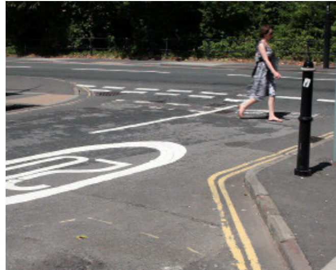
Fig.73 In some circumstances, when speeds on priority roads are relatively low and flows comparatively light, it may be acceptable to reduce the radii of kerbs at junctions to slow down traffic and make crossing easier for pedestrians. This should be informed by the Place and Movement functions of the streets.
