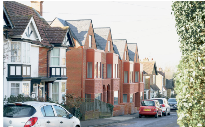
Street hierarchy within a suburban context - Keelson Yard by 31/44 Architects © Nick Dearden
